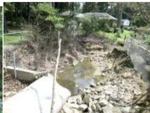
Outlet of Yarmouth Dr Culvert
