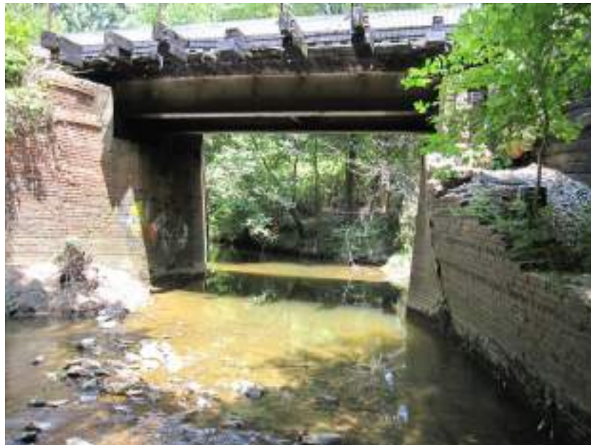
Figure 12. Railroad Bridge over Kinley Creek looking D/S (USACE)
