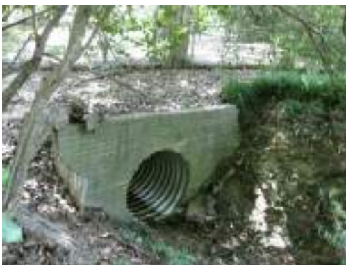
Inlet to Yarmouth Dr Crossing
