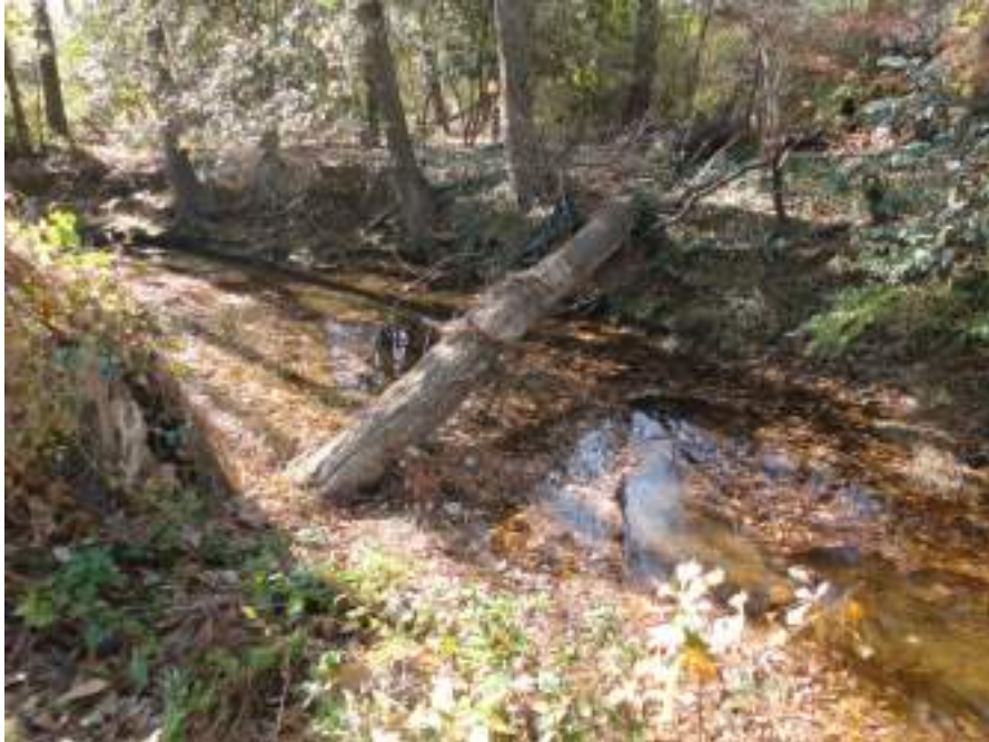
Fallen Tree in Kinley Creek and multiple trees with exposed roots along Kinley Creek.
